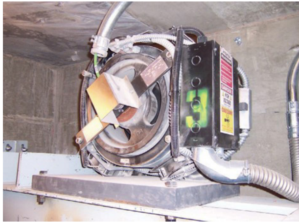
Figure 1: MRL driving machine; image courtesy of Delaware Elevator Co.
