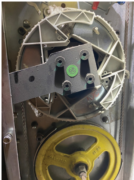
Figure 6: Car-mounted governor
