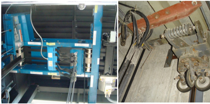
Figure 2: Governor (image courtesy of Otis Elevator Co.); safety (image courtesy of Richard Baxter)
