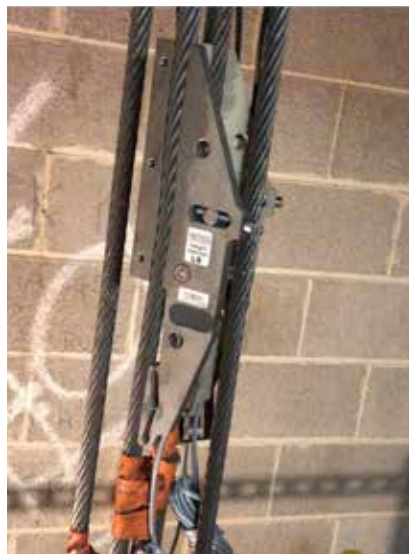
Figure 2: Henning LS1 rope gauge
