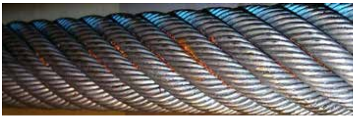
Figure 2: Rouge can be seen between the rope strands here.
