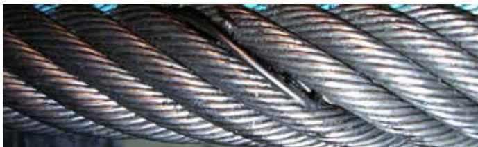
Figure 3: A valley break is visible here. Any breaks not at the top (crown) of the wire are internal and indicate extra concern for internal (unseen) rope condition.
