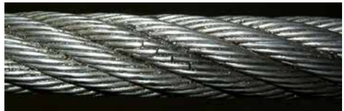
Figure 7: Four wire breaks side-by-side. The maximum permitted is 16 per lay in normal wear conditions and eight in unfavorable wear conditions.
