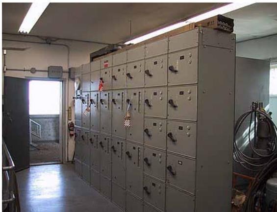
Motor control center with disconnects for multiple 480-V motors. The terminations, if improperly torqued, can overheat and cause an electrical fire.
