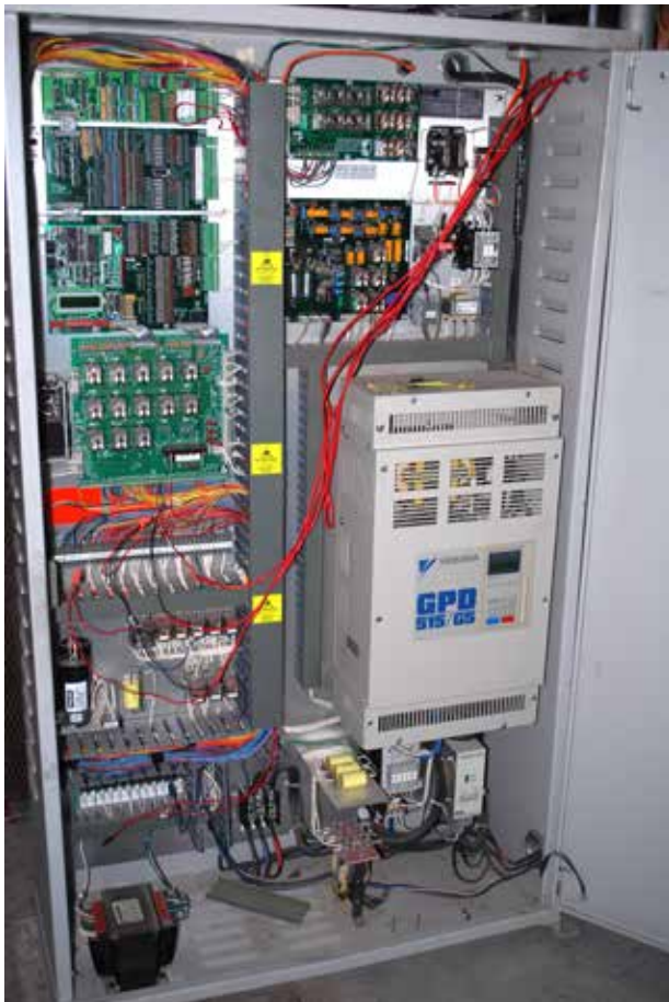
The elevator motion controller feeds data to the VFD inverter section.
