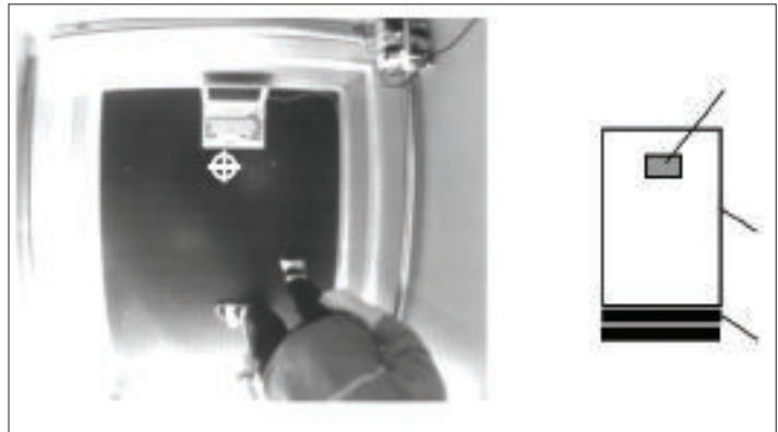
Figure 3: Incorrect mounting location for ESPROS/VOL-V in ceiling of elevator cab (0.5 m from back of elevator cab)
