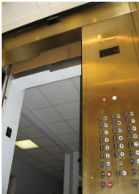
CEDES ESPROS/VOL camera installation (photo courtesy of New York Elevator)
