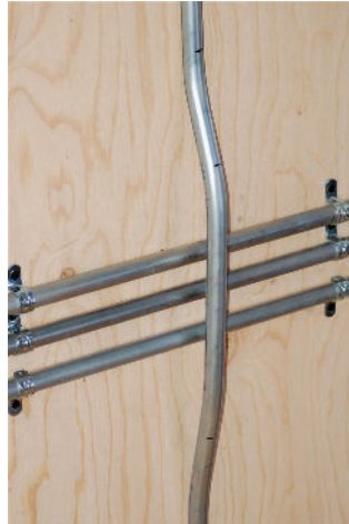
Figure 2: A four-point saddle bend is used where two or more pipes must be traversed.
