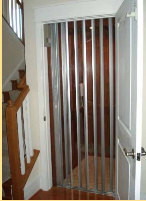
Figure 4: Accordion carriage gate; photo courtesy of Atlantic Elevator
