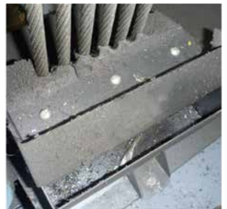
Figure 9: A case in which an automatic rope lubricator’s felt is poorly aligned and worn, and the reservoir is dry.
